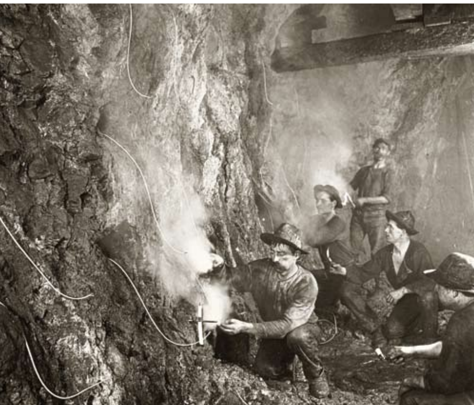
FIGURE 15.6: Miners set dynamite to loosen underground rock. They had to figure out how to blast just enough rock to keep up production without causing a cave-in—which inevitably killed people.
