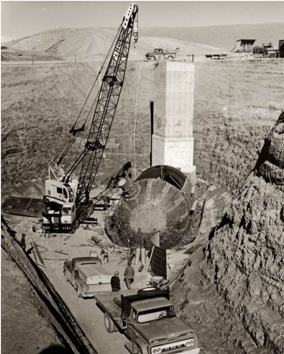
FIGURE 20.12: After the Air Force built the intercontinental ballistic missile silos and launch sites, they buried them deep underground. The Air Force chose Montana for the silos because of its high elevation (which reduced the altitude the missiles had to climb) and stable soil structure. In addition, the state's sparse population made it a more acceptable target if the Soviets attacked the missile sites.
