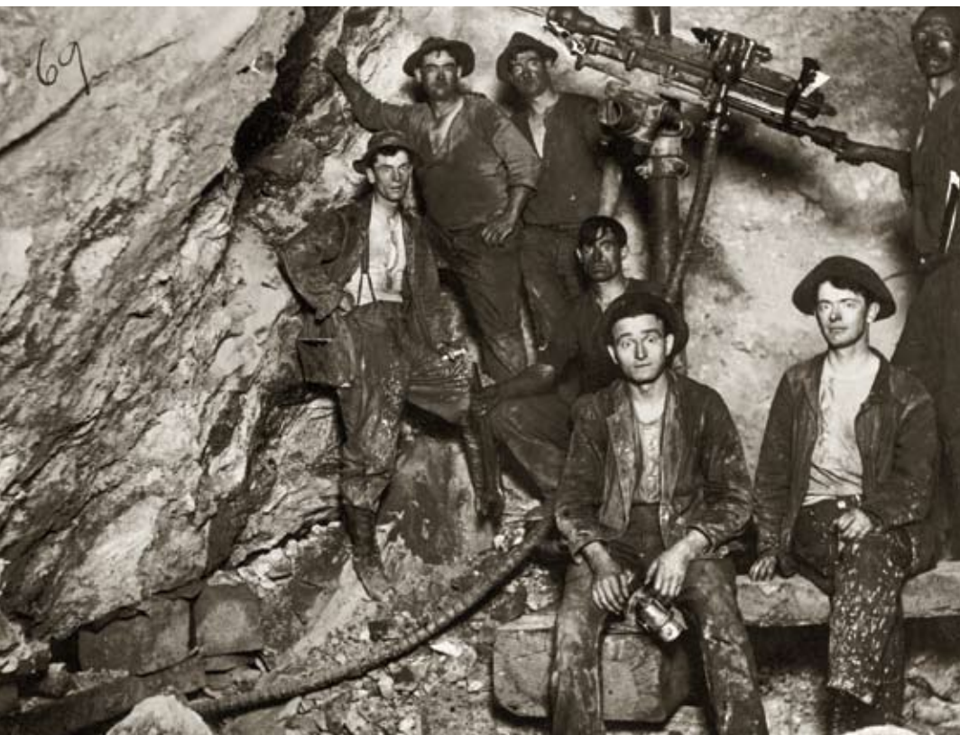
FIGURE 16.6: Machine drills increased productivity, but they also filled the mine tunnels with fine rock dust that scarred miners' lungs. Miners called the machine drills "widowmakers" because they caused so many miners to die from lung disease.
